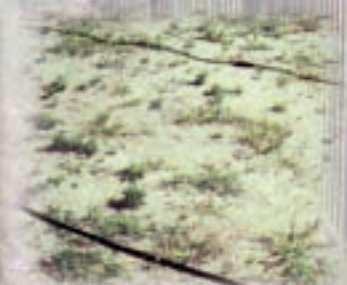
Cable to Cable Installation
