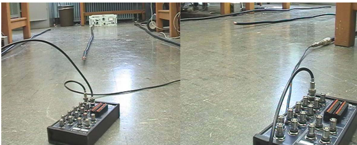
Figure E2: Left: Typical setup of the three LCX system. Cables are placed 1m apart with the tLCX in the center. The cables are each 11feet in length, terminated by two 100 \Omega resistors soldered between the inner and outer conductor. Right: N type-BNC adaptors were attached to the rLCXs. A standard 50 \Omega probe connected the cables to the 2110. Note: The 2110 is free from the computer for demonstration purposes.
