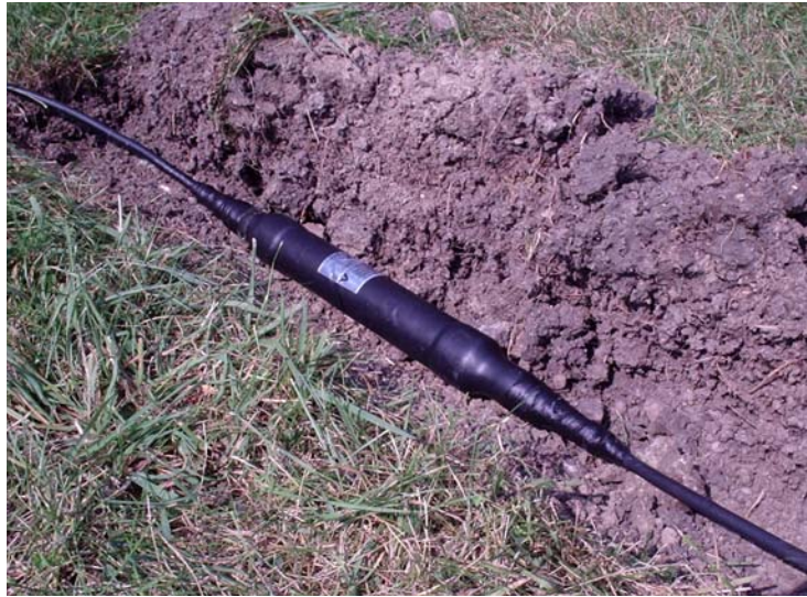
Fig. 1 -burying a transmitter
